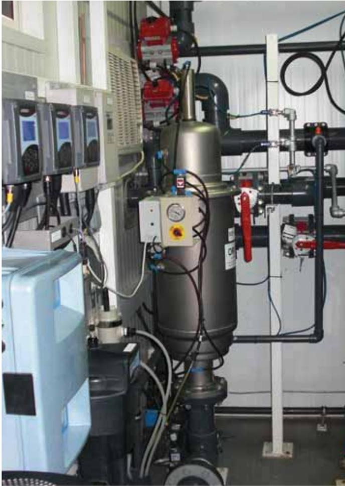
TSE Wet Well Pumps → Pre-Chlorination Dosing → Coagulant Dosing → MF Feed / Backwash Pump → MF Self Cleaning Filter → Micro Filtration Unit → Filtered Water Tank → RO Feed Pump → Ultraviolet Unit → Cartridge Filter → Acid Dosing → Antiscalant Dosing → SBS Dosing → RO High Pressure Pump → Reverse Osmosis Unit → Discharge Water Tank → Wet Well
