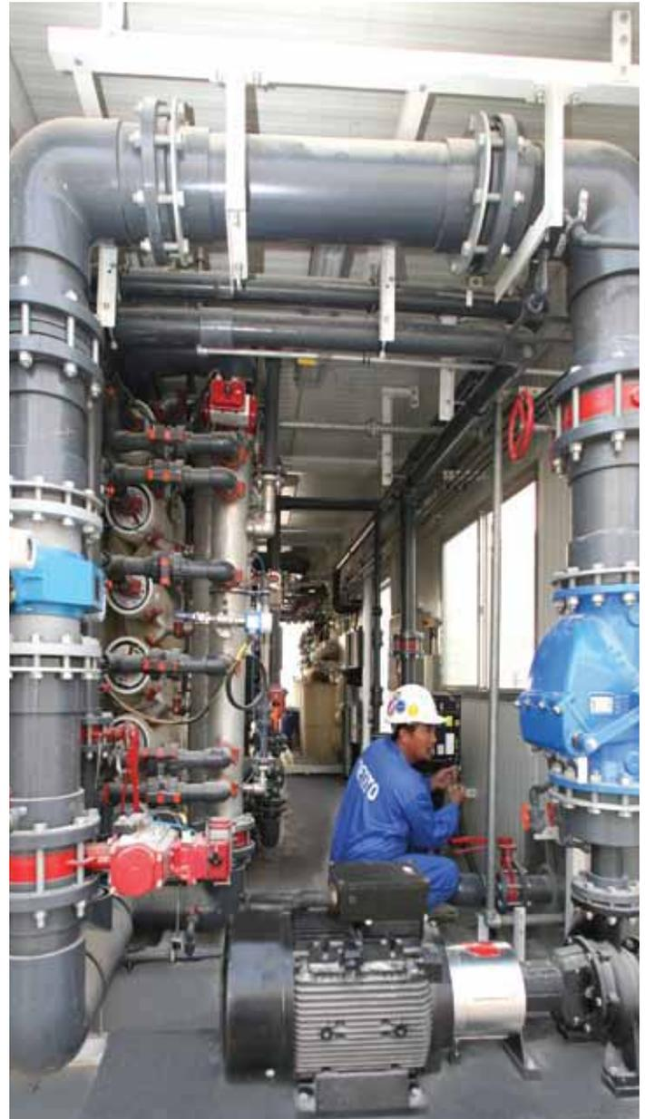
Feed water from the TSE wet well is delivered to the buffer tank via submersible pumps. The buffer tank acts as a steady source of water to the two filtration units running in parallel. Filtrate and product water are lead back to the TSE wet well. Water containing chemicals in high concentration, i.e. UF and MF chemical backwash water, is collected in a chemical waste holding tank where it is neutralized and sent back to the TSE wet well.
