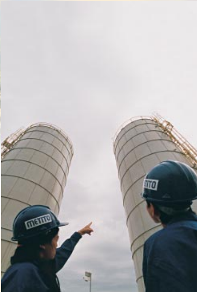
TOWERING LIME SILOS HOUSING LIME SLAKING & SOLUTION TANKS
