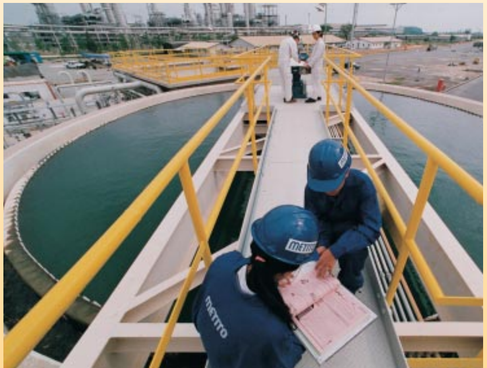
GENERAL VIEW OF WATER PRE TREATMENT UNITS
