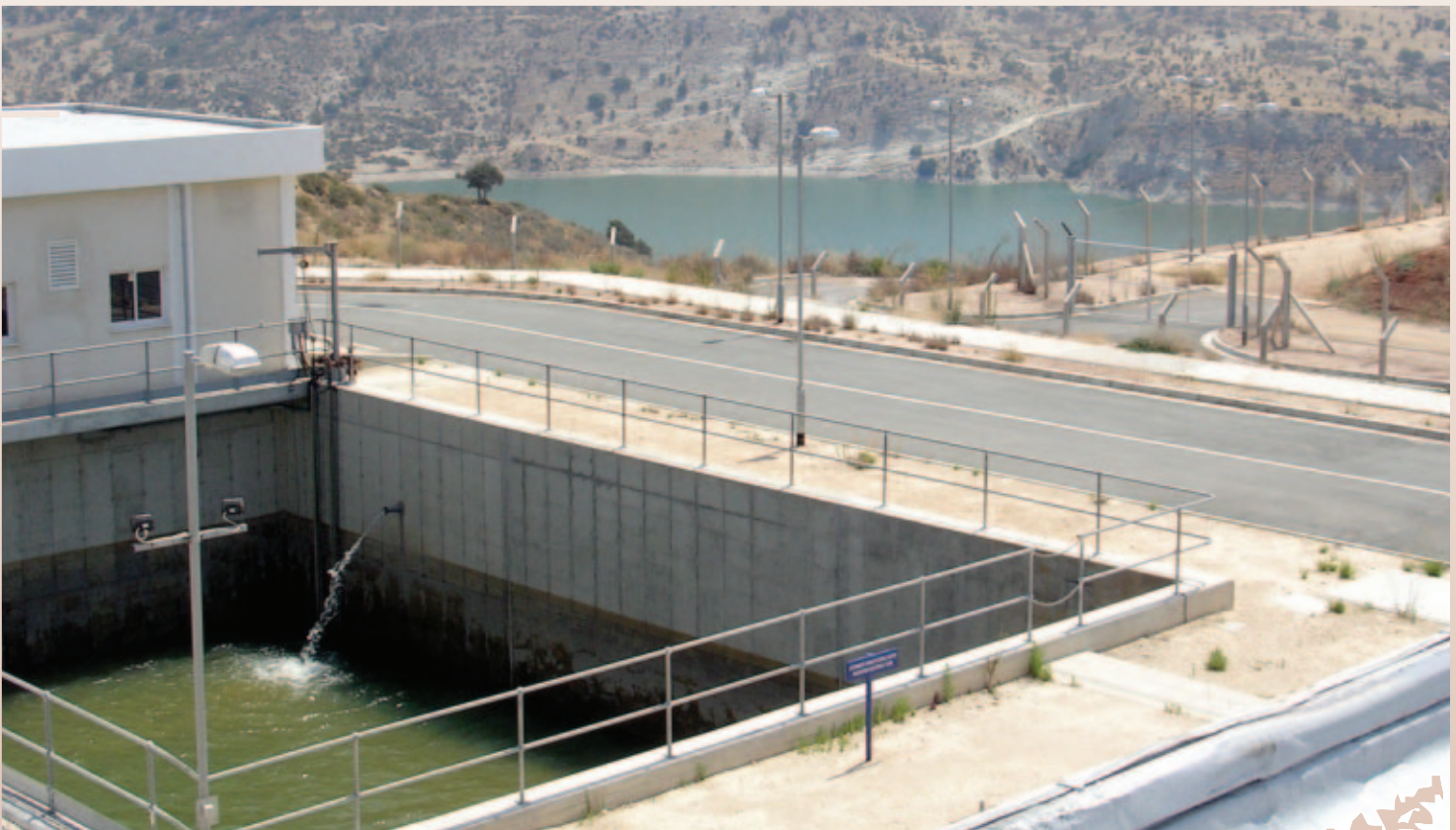
AN OVERVIEW OF THE WATER TREATMENT PLANT SITE
