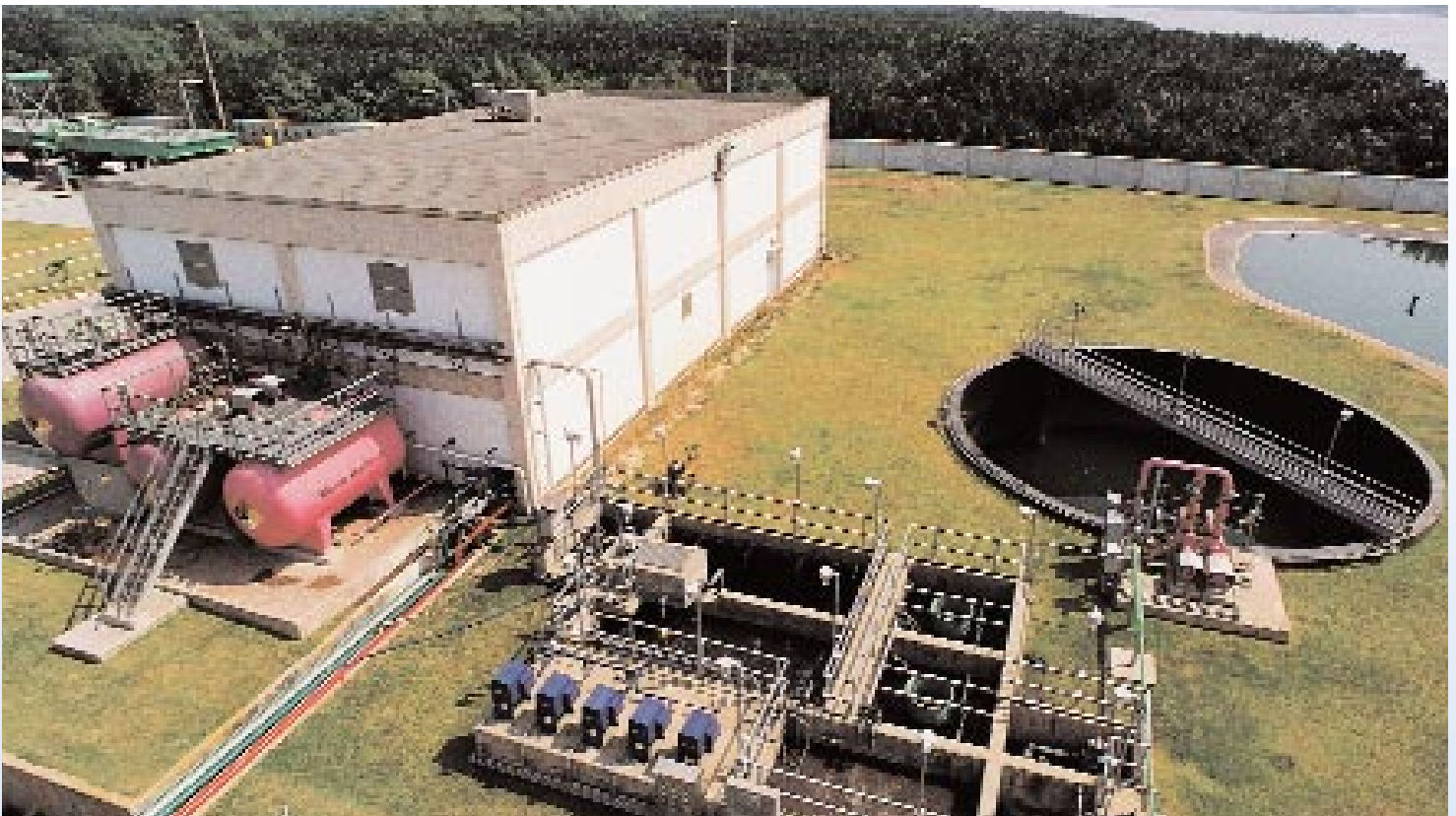
View of the demineralization plant building, sewage and waste treatment plant
